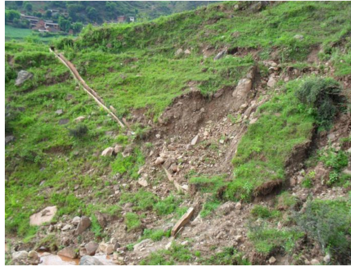
Fig. 4. Partial collapse of front edge of Guanzhuangdian landslide
